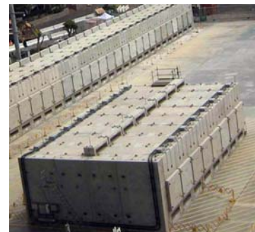
San Onofre's dry cask storage facility
